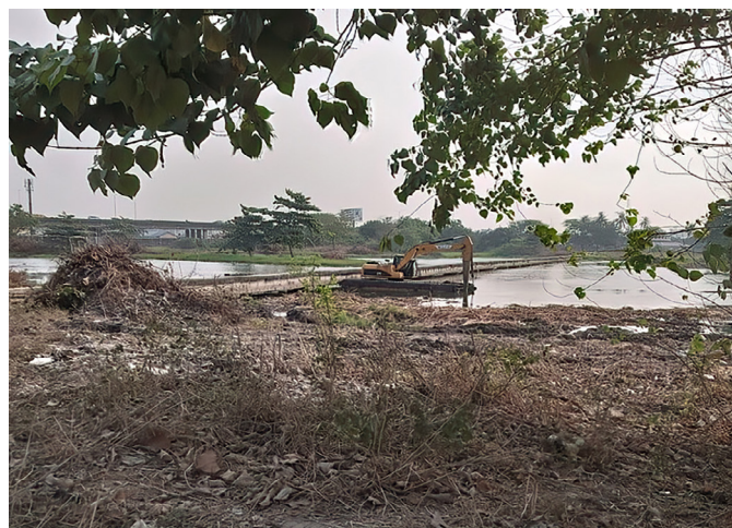
Destruction of vegetation at wetland site
