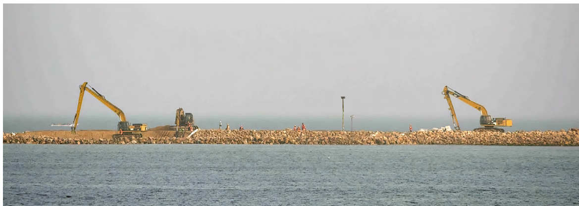
Construction of a new port at Popenguine on Senegal's Petite Côte
